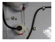
Step 5: Fit O-ring to bottom of Quartz sleeve as shown then screw bottom nut tightly onto chamber using your hand.
